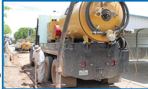
Crews are shown installing buried fiber optic cable in the Pueblo addition in Dalhart.
